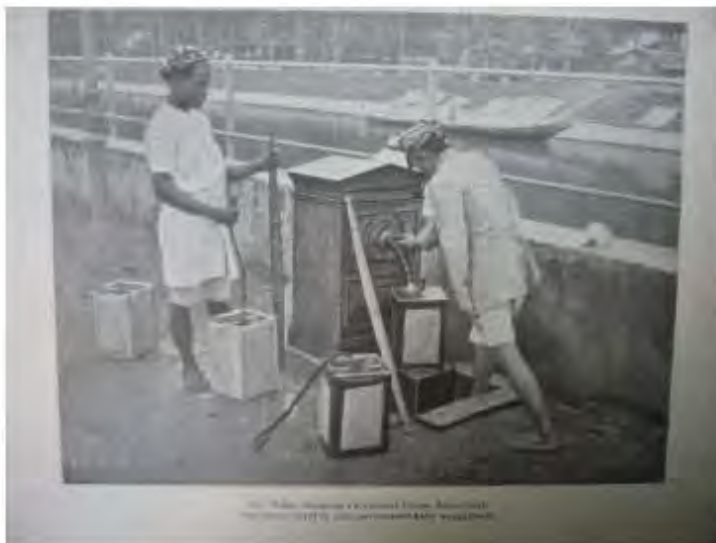
Taking water from the hydrant Passar Baroe-East The water is hauled in petro-cans
